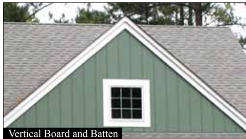
Vertical Board and Batten
