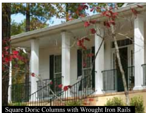
Square Doric Columns with Wrought Iron Rails
